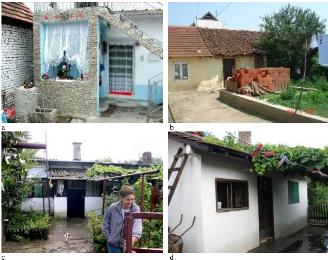
Photo 3 SELF-HELP CONSTRUCTION OF HOUSE
