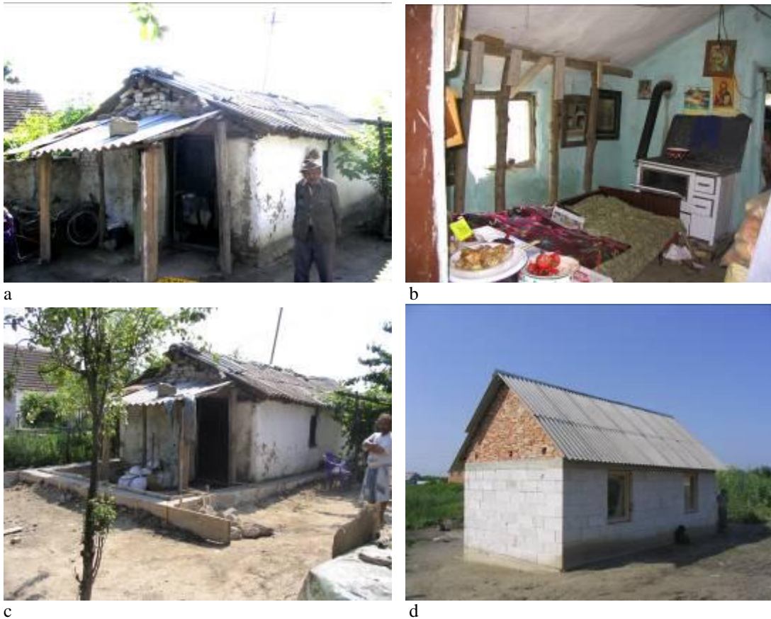
Photo 12 BUILDING A NEW HOUSE ON THE SITE OF THE OLD ONE
