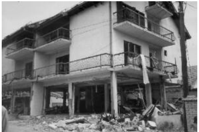
Urosevac: the former OSCE-KVM office building, which was mined and blown up [zoom]
