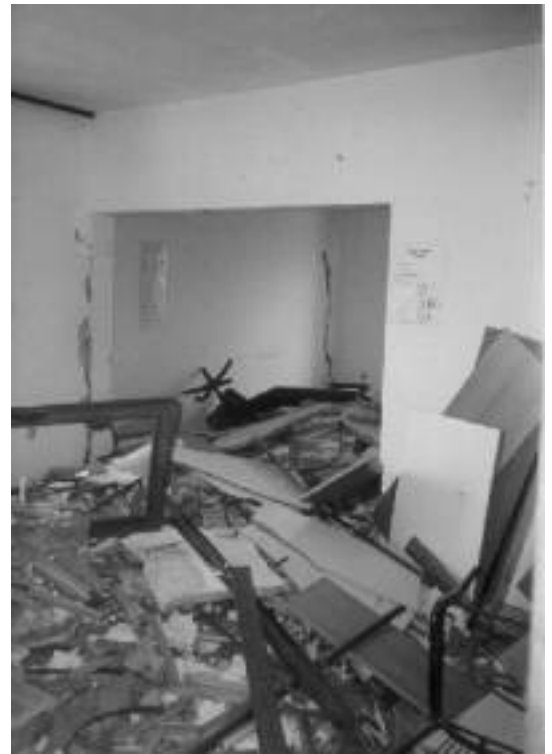
The OSCE-KVM Co-ordination Centre (Urosevac/Ferizaj), after it was mined and blown up [zoom]
