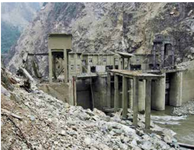
Figure 39. Damaged Gengda Hydropower Plant (left) and nearby substation (right) near the epicenter of the Wenchuan Earthquake (Photo credit: Mingchong Liu).
