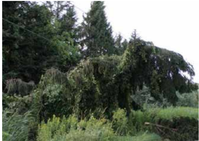
Figure 24. Power line damages caused by wind throw.
