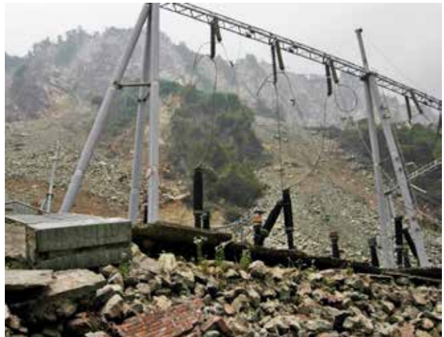
Figure 39. Damaged Gengda Hydropower Plant (left) and nearby substation (right) near the epicenter of the Wenchuan Earthquake (Photo credit: Mingchong Liu).
