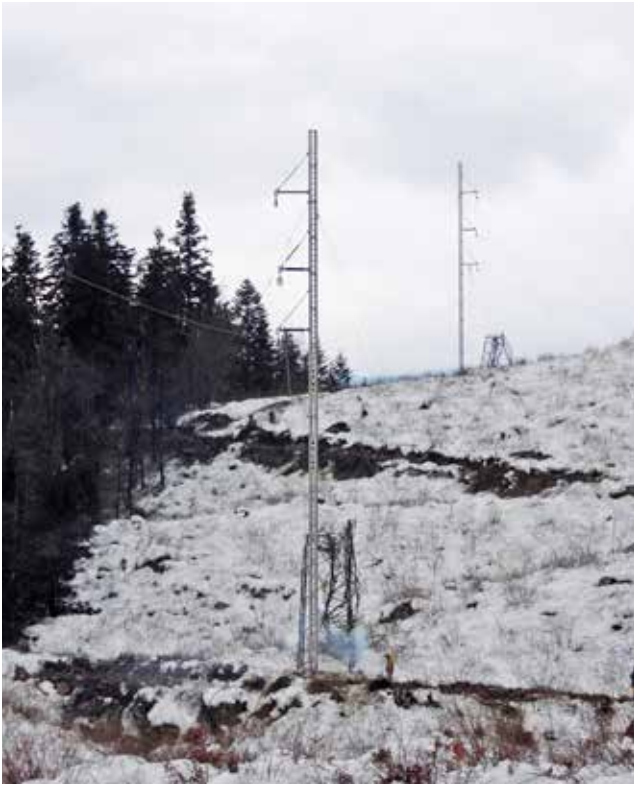
Figure 32. Emergency restoration structures (ERS)
