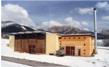
District heating plant
