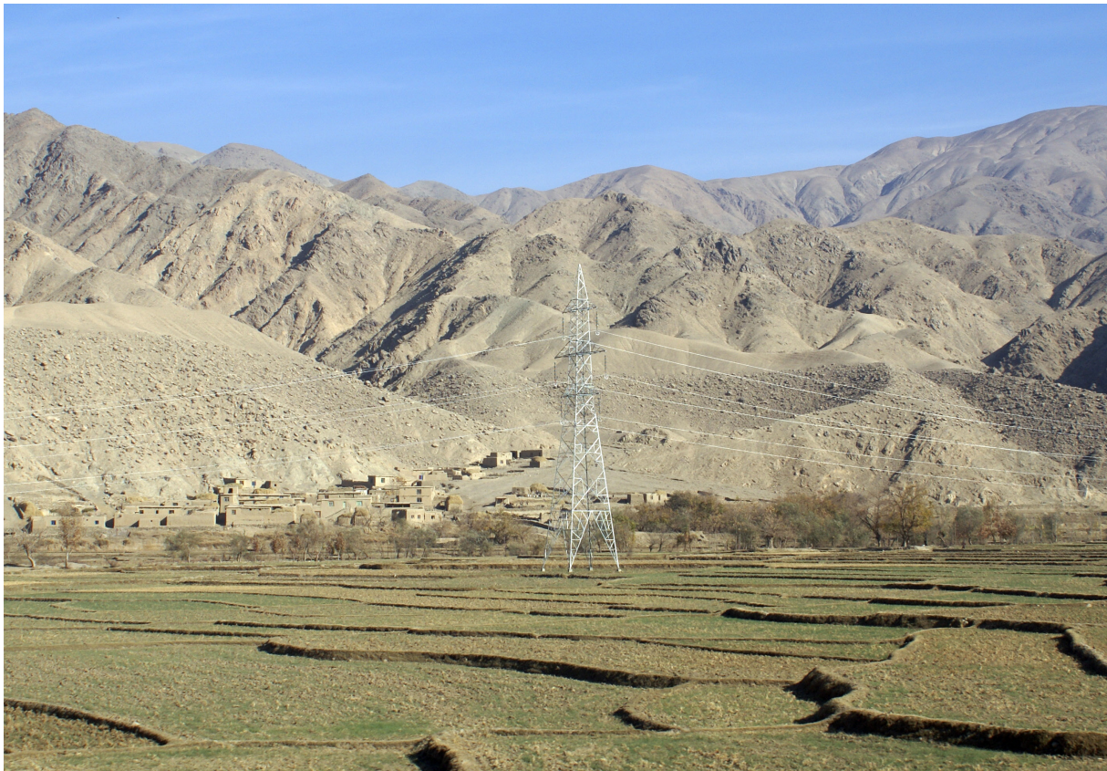
© Zoi Environment Network Power infrastructure in northern Afghanistan
